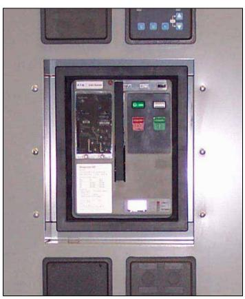
Figure 12. Insulated Case Switching Device.
